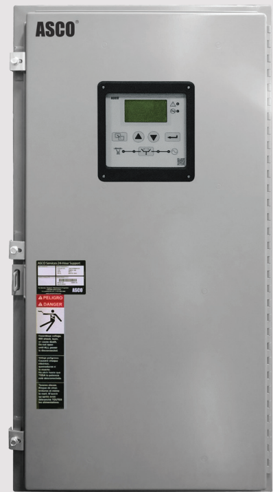
Figure 2: A non-secure, single-door, Type 3R enclosure. The controls are exposed to the environment and accessible to anyone.
