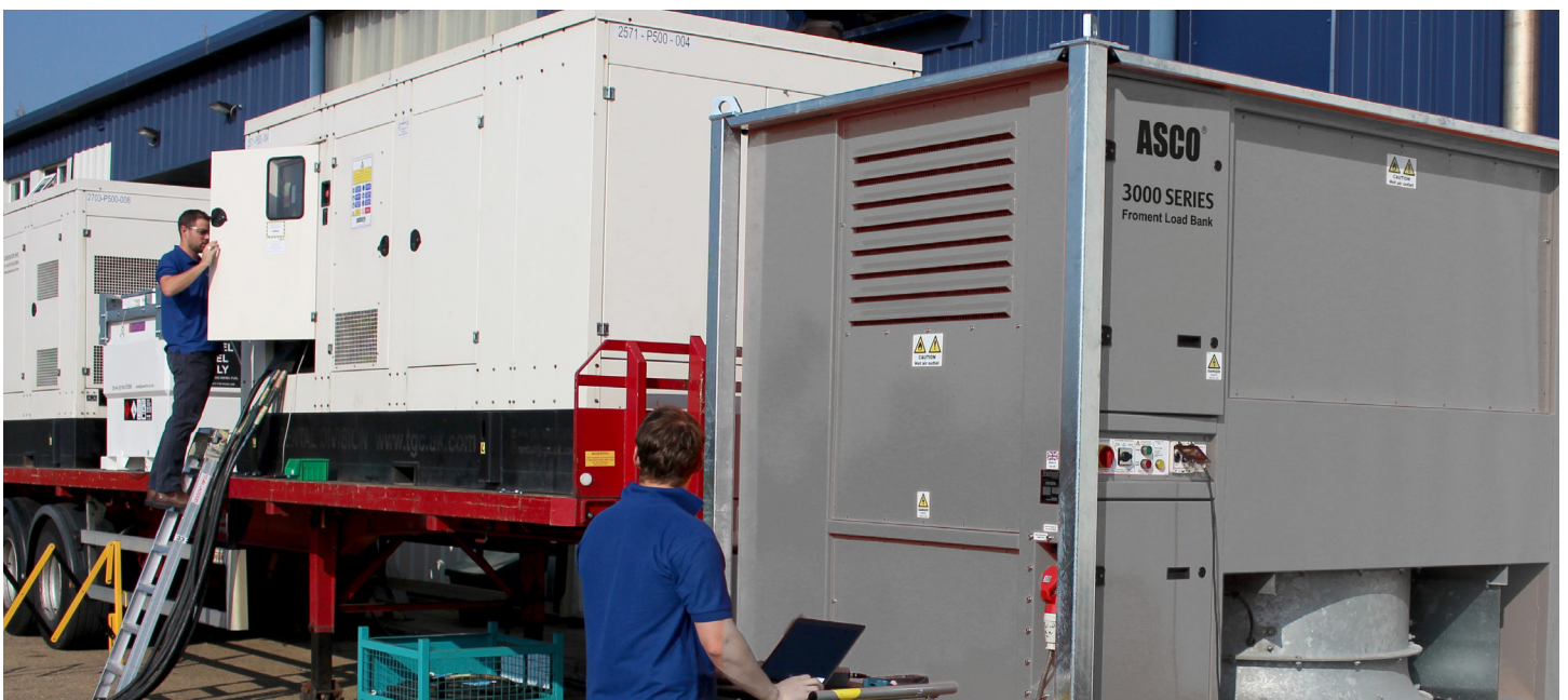
Load testing two diesel generating sets in parallel
